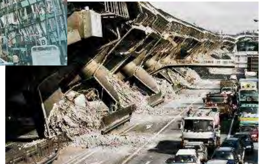
Collapsed viaducts of an expressway
